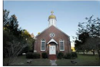
Sts. Peter and Paul Russian Orthodox Church in St. Helena, a town about 10 minutes south of Burgaw, is deteriorating. Its membership is down to four people, and there is no resident priest for Masses.
