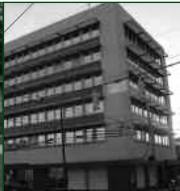
Tide Water Power & Light Building, 320 Chestnut Street, Wilmington, NC.
